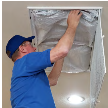
5. Close off the return side of air handler by putting a filter in a plastic bag and reinstalling it into its holder.
