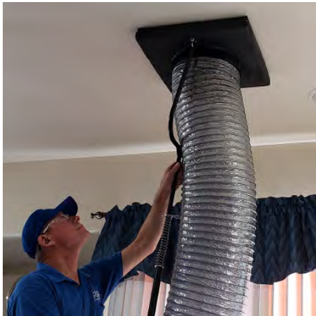
4a. Connect the other end to the most effective supply duct location using the optional Pogo Pole hose adapter or adapter plate.
