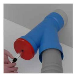
6) Turn on the vacuum motors in the Air-Care DuctMaster then insert the 4" brush into the dryer vent. The drill will not run unless BOTH the trigger switch in the drill handle and the foot pedal are turned ON, Start the drill using the foot pedal only AFTER the brush has been inserted into the duct.
